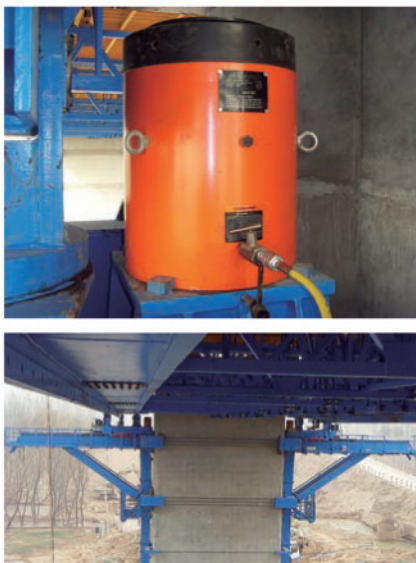
400 ton EAGLE PRO EL series hydraulic cylinders used in bridge building
